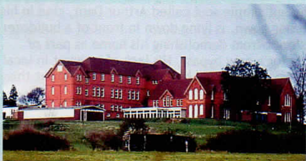
The Police Cadet School and College at Priory Park before demolition
