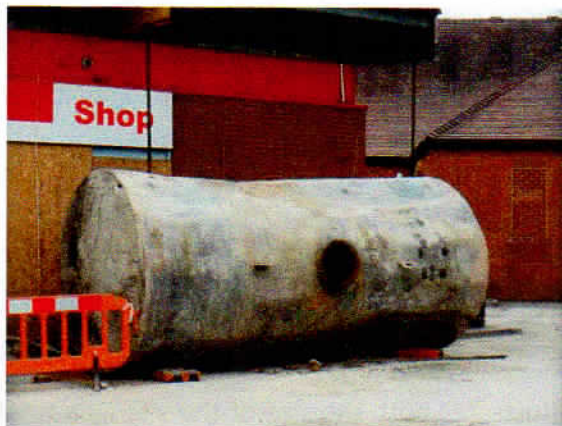
One of the large petrol tanks after its removal
